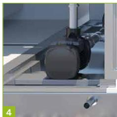
Rotary pump in redundant design
